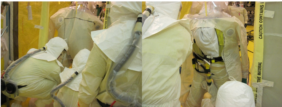
Figure 1: Employees developed a method to cut workers out of Level B suits by marking cut lines on the backside of the suits and applying tape over the cut lines prior to use keep the cut lines free of contamination. During doffing, a support crew cuts the back of the suit away from the worker, allowing the worker to step backward out of the suit.
